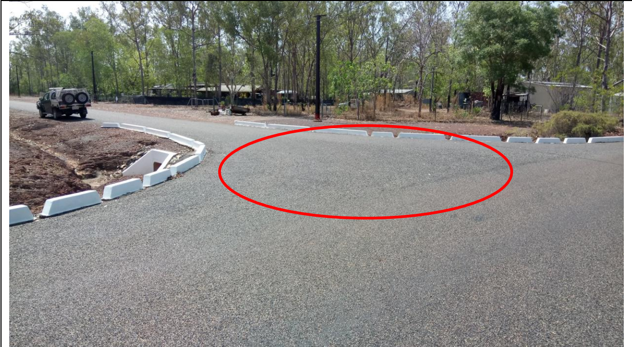
Ravelling at Kathleen Circuit Intersection
