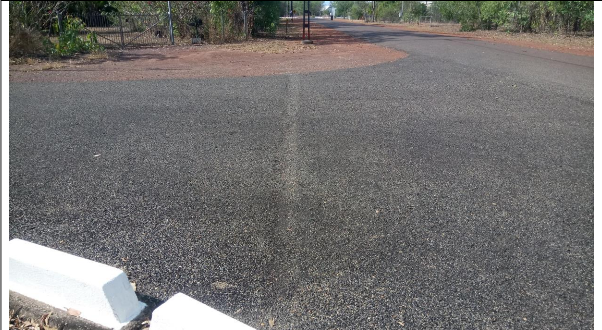
Service Crossing adjacent to Baluria Road
