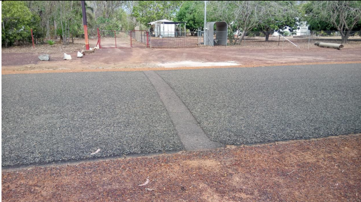
Service crossing at CH0.3
