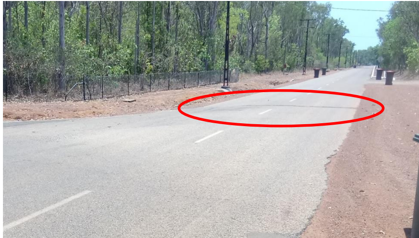
Service crossing Dalmeny Street
