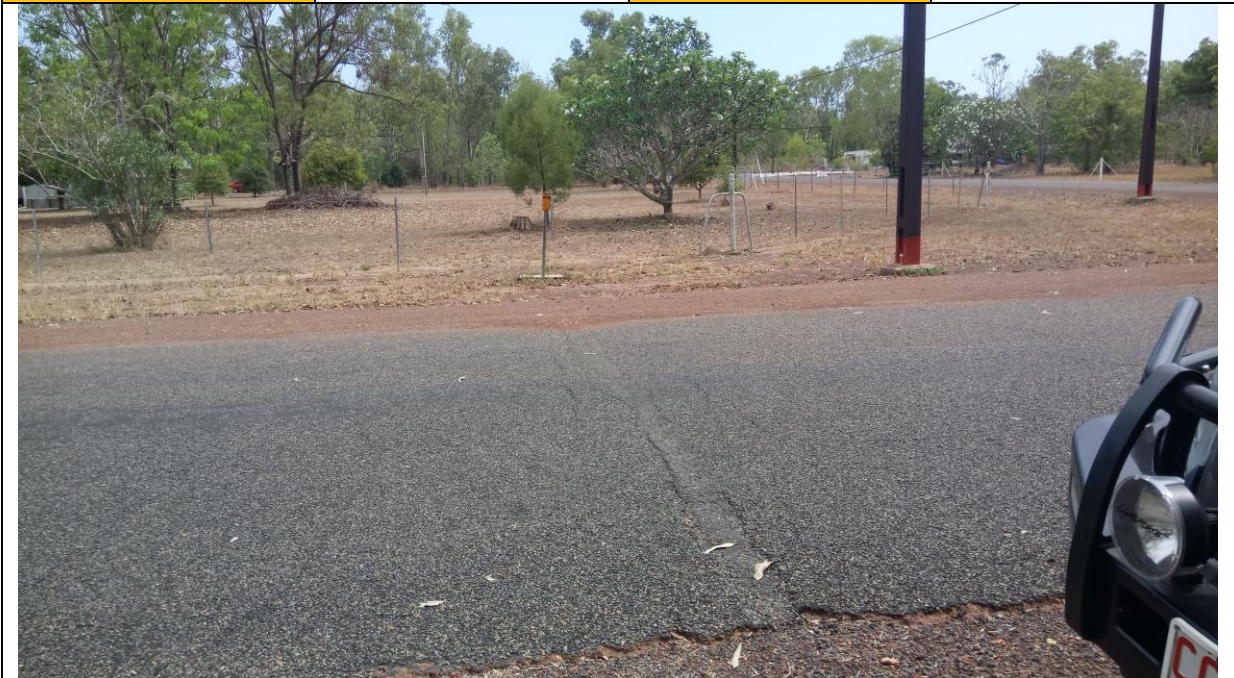
Service Crossing near Baluria Road Intersection
