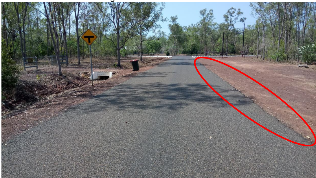
Edge break between CH0.4-0.5
