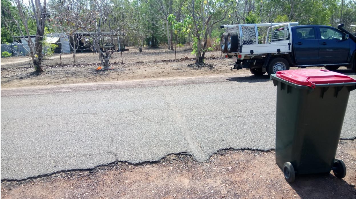
Service crossing at approximately CH0.75
