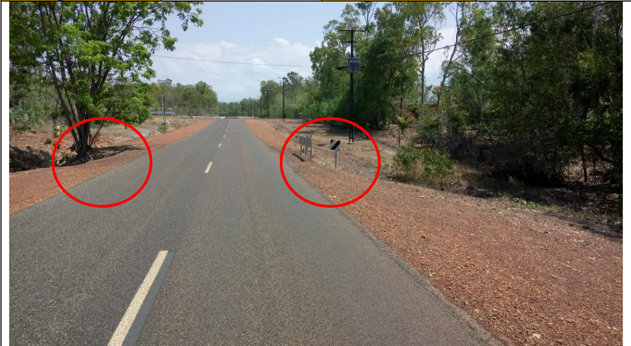
Culvert approximate chainage 0.45
