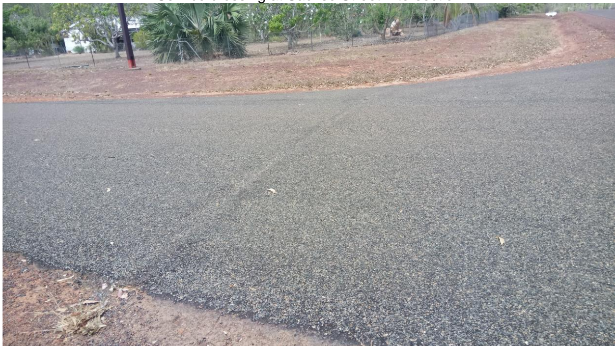
Service crossing at Milady Street Intersection
