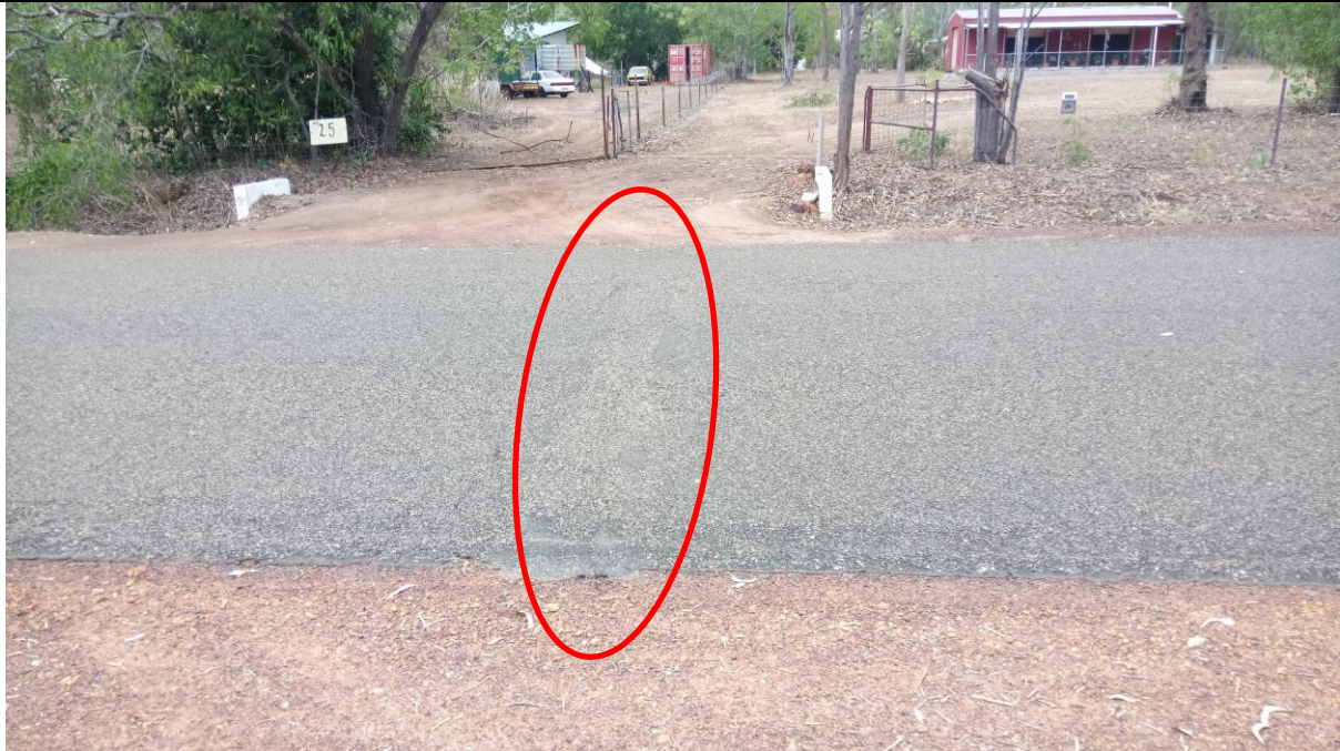
Service crossing approximate chainage 0.35
