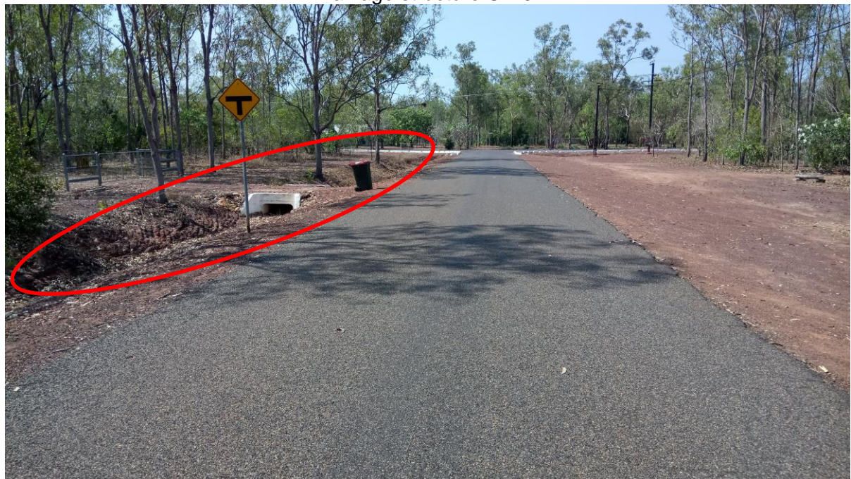
Drainage structure CH0.4
