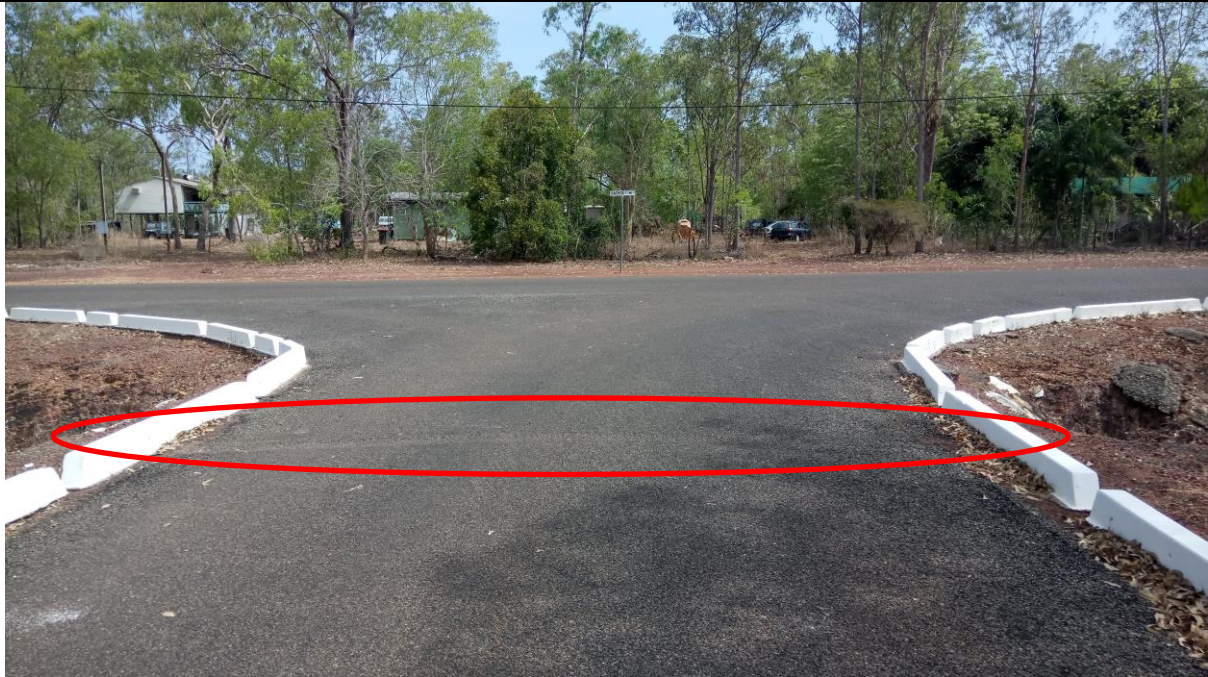
Service crossing at Sachse Street Intersection
