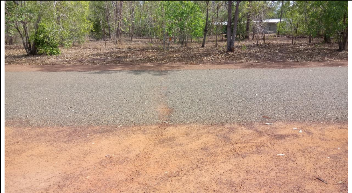
Service Crossing approximate chainage 0.15
