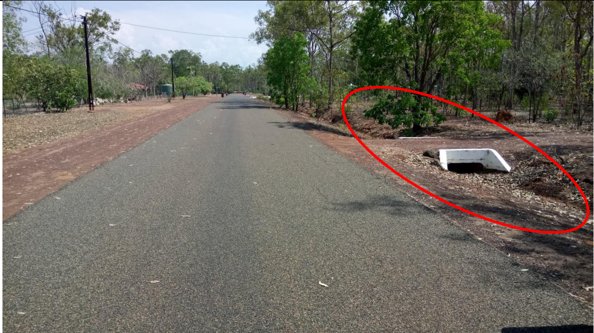
Drainage structure CH.02
