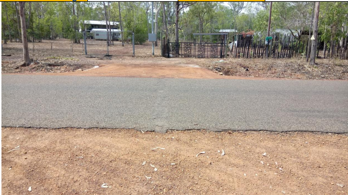
Service Crossing approximate chainage 0.35
