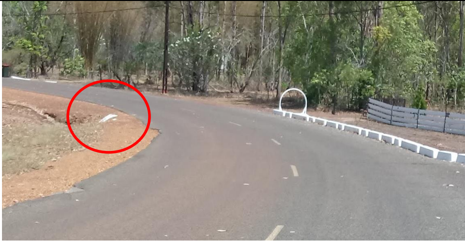
Culvert approximate chainage 0.95
