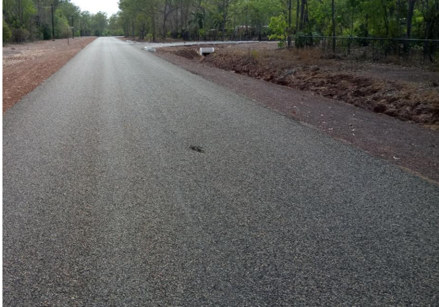
Pothole approximate chainage 0.2
