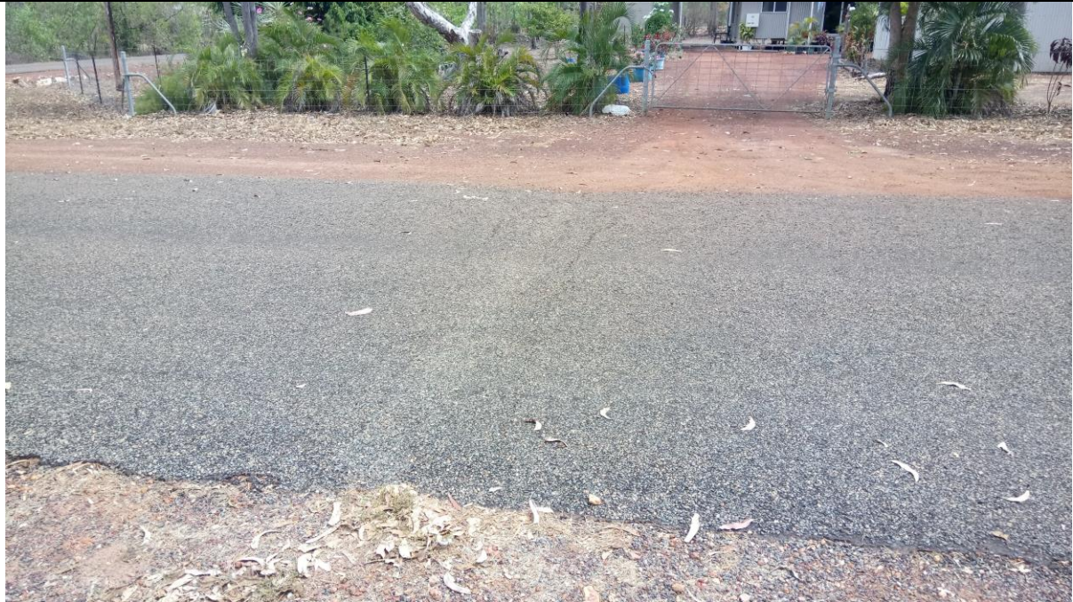
Service crossing approximate chainage 0.15
