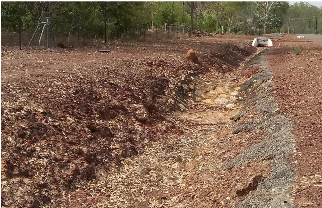
Photo: Example erosion protection Massey Street
