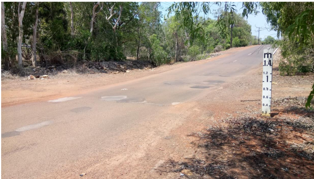
Photo: 92 Cox Drive
