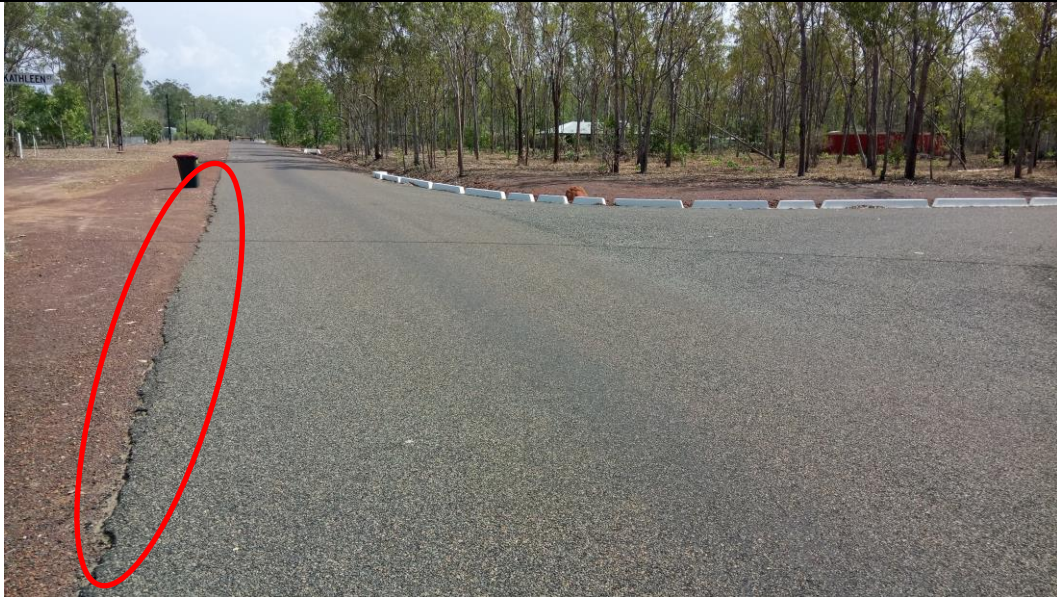
Edge Break between CH0.2-0.3
