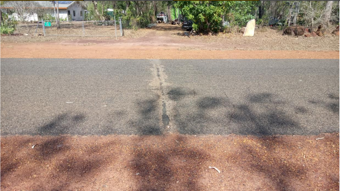
Service crossing approximate Chainage 0.25
