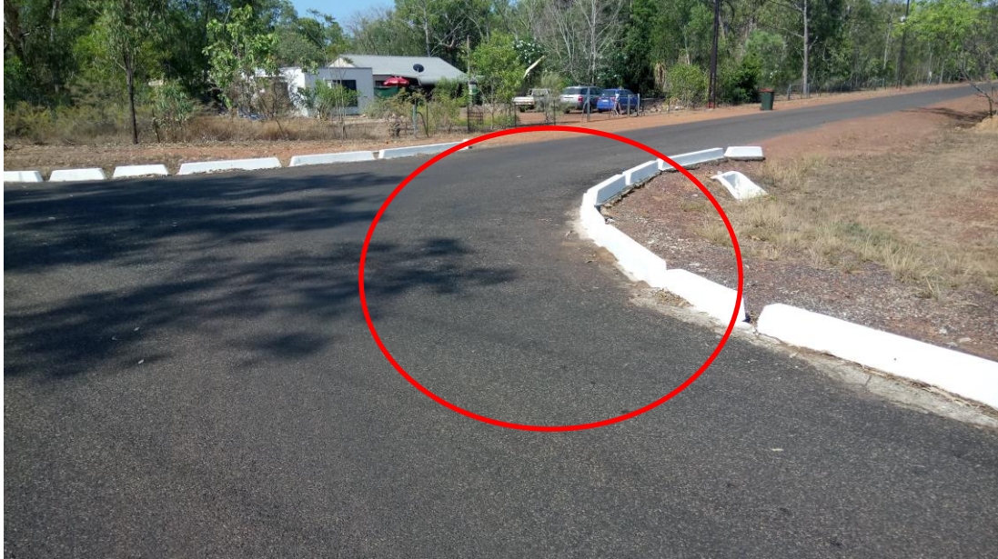
Ravelling Uhr Road Intersection
