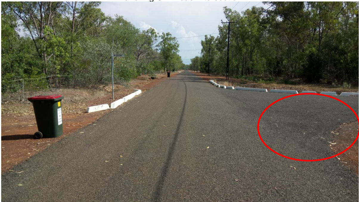
Ravelling Boom Place Intersection
