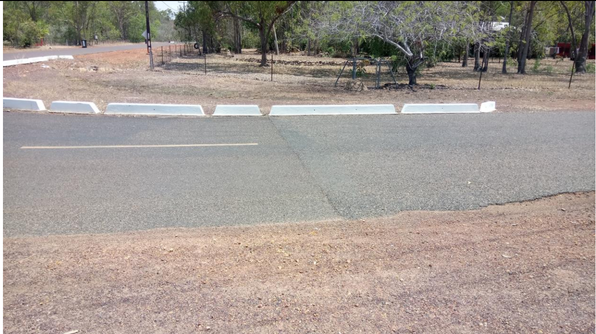
Service crossing adjacent to Baluria Road Intersection
