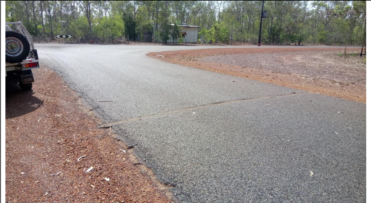
Service crossing approximate chainage 0.55
