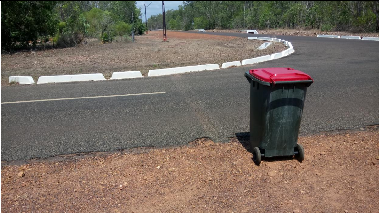
Service crossing Sachse Street Intersection
