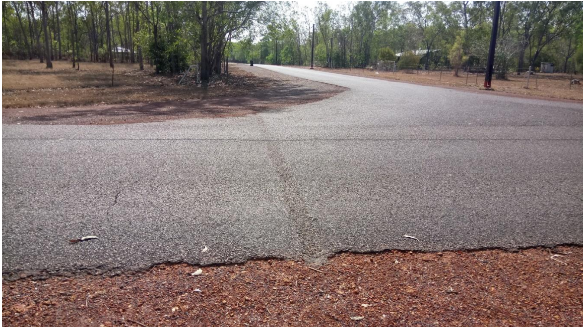
Service crossing adjacent to Sachse Street
