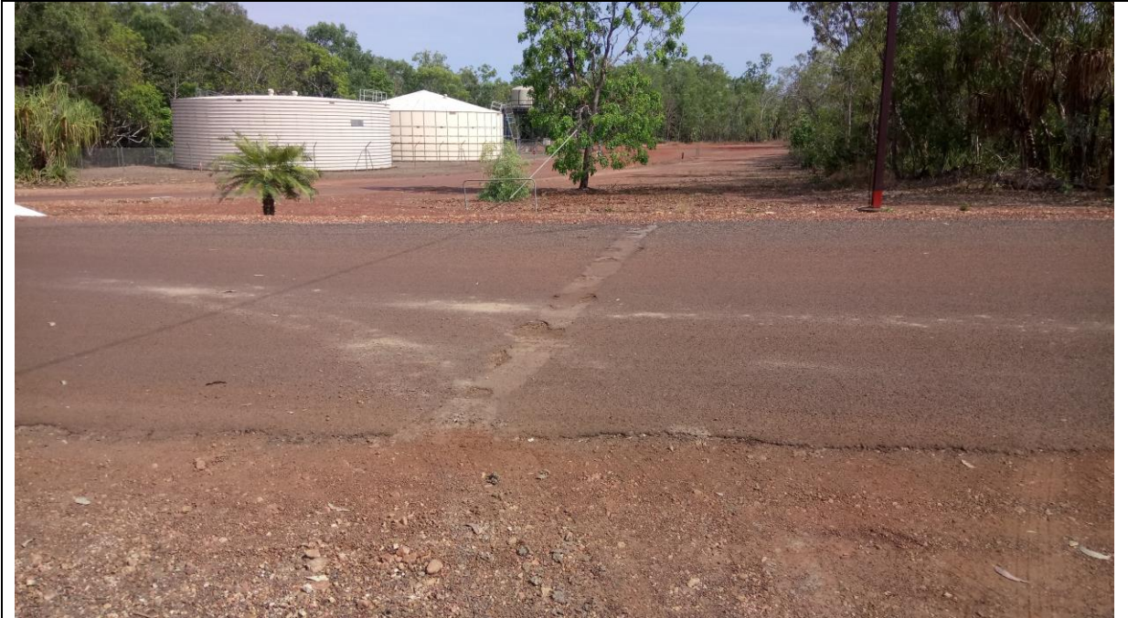
Service crossing approximate chainage 0.15
