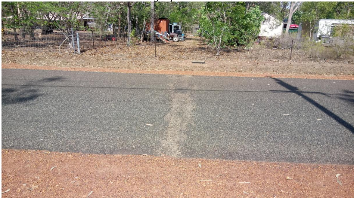
Service Crossing approximate Chainage 0.9
